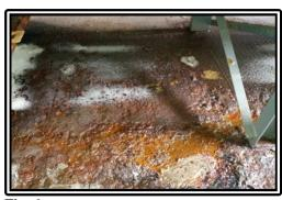
Fig. 6 Corroded floor at DB2 Terminal
