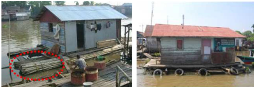
Figure1. Bamboo foundation and semi-fixed element “tire” as protection for foundation still in place Source: Dahlani et al, 2015
